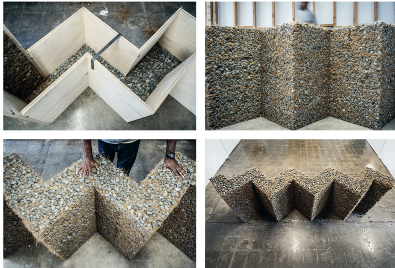
A zigzag wall was built with only loose rocks and coconut husks using a slip-forming method to promote granular jamming in a fast, efficient, and reversible manner. Credit: Self-Assembly Lab, MIT, Google
